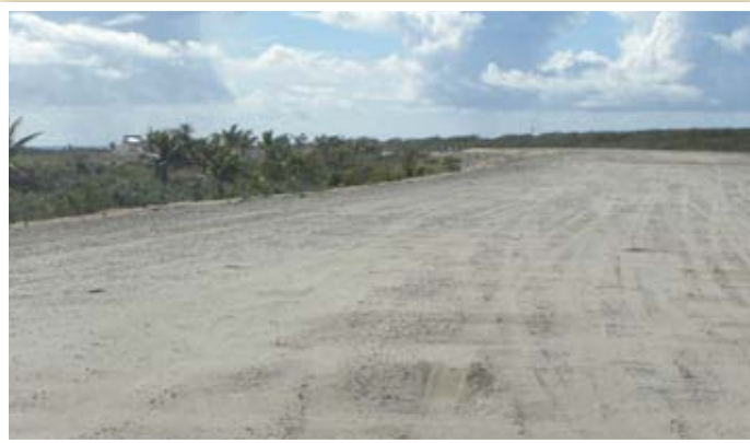
THE COMPLETED SECONDARY DUNE SYSTEM.
