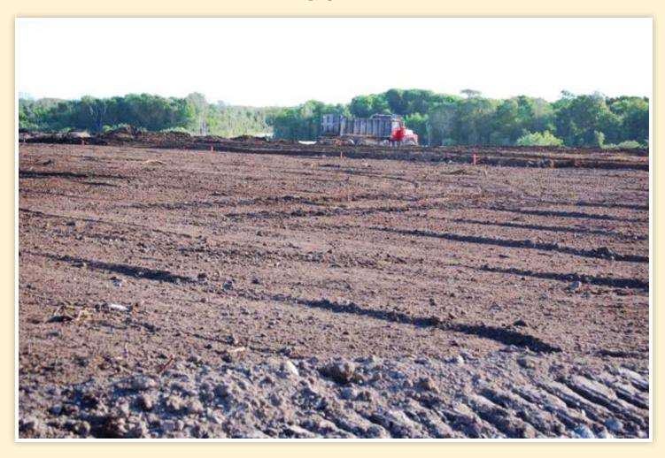
All buildable lots are currently being covered with two feet of dark, rich topsoil that has been sourced exclusively onsite. The soil has been washed and filtered using groundwater from the harbour project and will prove a rich bedding compound for grass, trees, flowers,
